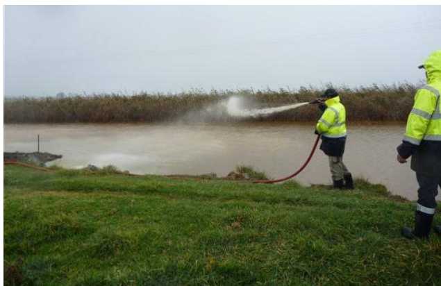
Figure 2. Limestone dosing undertaken by the EPA
