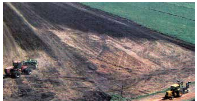
Laser levelling on the Lower Murray.
